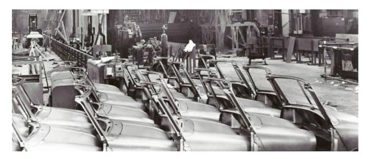
When BMC type cars were made in the 1950's to the 80's, the bodyshell would usually be made up from sub-components, often from different factories. Each main component had a serial number attached to it for internal use only, usually on a welded-on steel plate with embossed numbers, about 0.5" high
